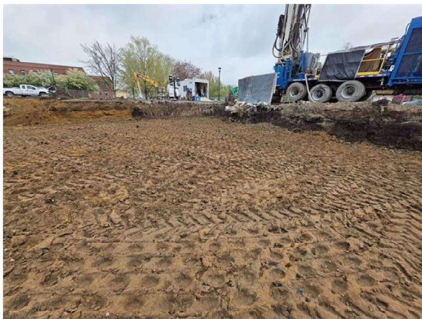
Compacted Structural Fill Placed
