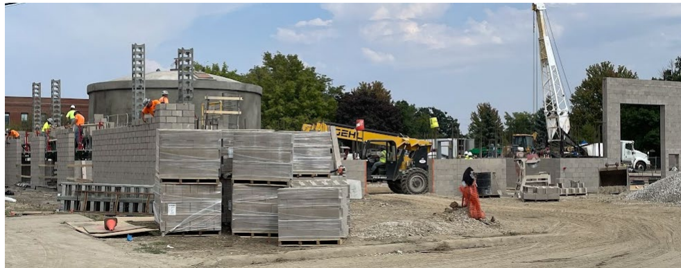
Crack in the existing detention tank and new water treatment plant under construction. Well #10 is near the white crane. The new concrete finished water ground storage tank is visible in the background to the left.
