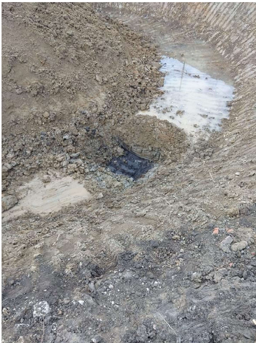
Soils below clearwell tank looking Southwest
