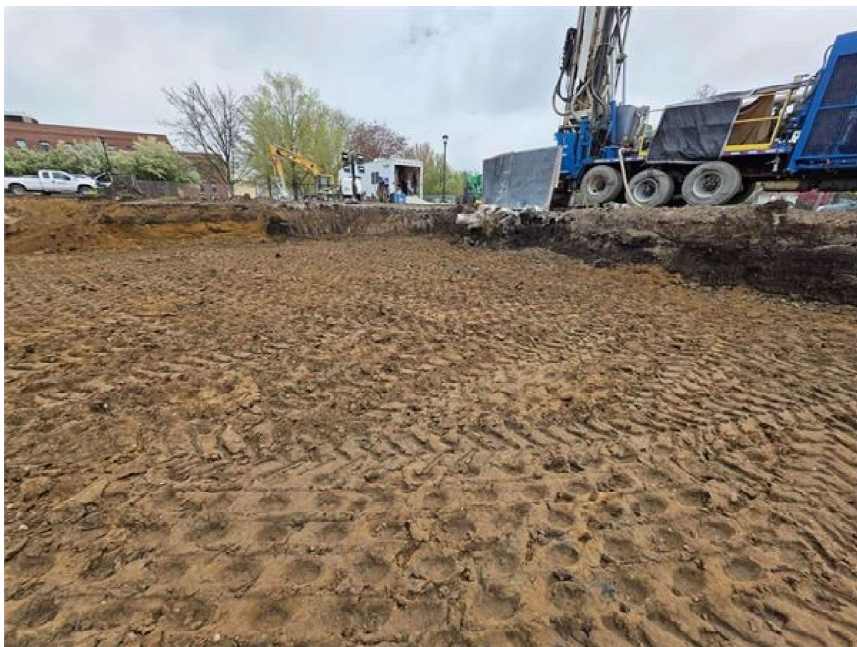
Compacted Structural Fill Placed
