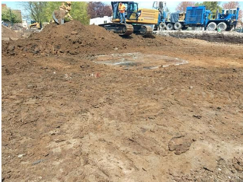
Concrete slab and cistern, looking Northeast
