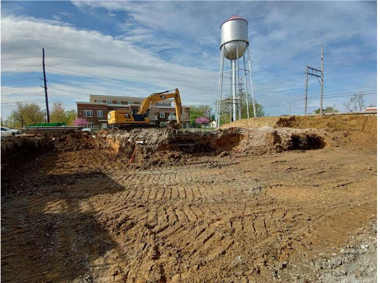
Photo 1. Area of Excavation Observation, Looking Southwest
