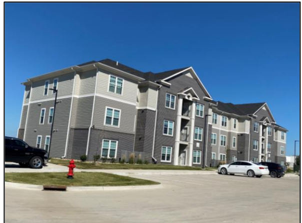
New construction multifamily rental building
