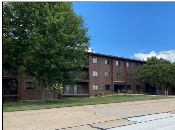
1980’s era owned multifamily (condominium) building
