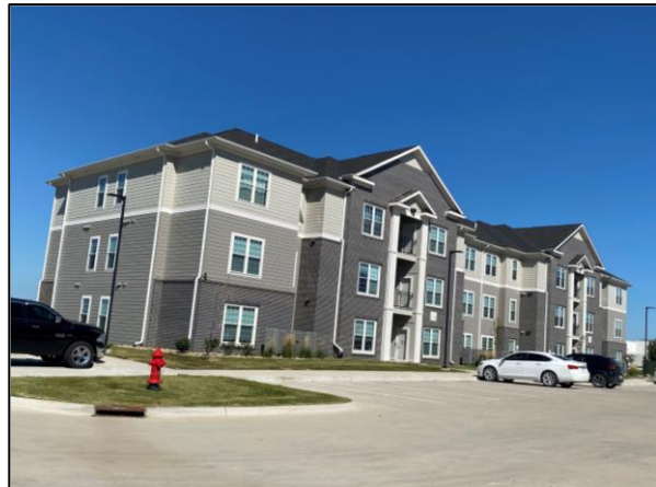
New construction multifamily rental building
